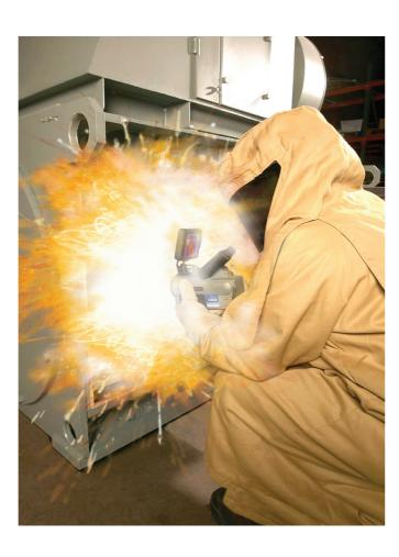
Most instances of arc-flash are due to the reduction of insulation and isolation distance between energized components, as commonly caused by:
